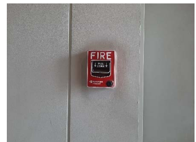
Fire Alarm Manual Station
