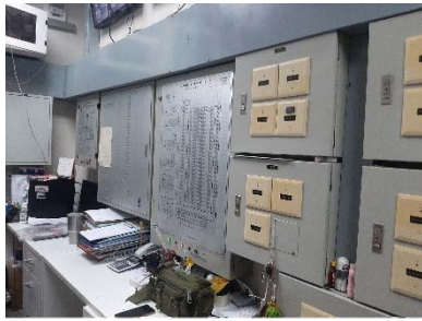
Graphic Annunciator Fire Alarm System
